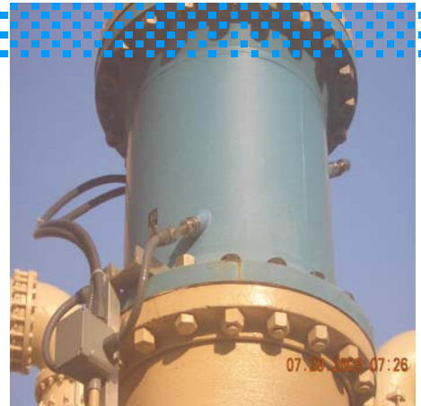
24" (DN600) 93C measures fresh water in Orlando, Florida USA after odorous hydrogen sulfide gas is removed.
