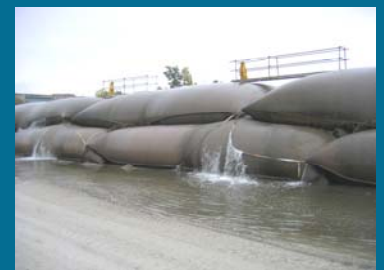
Weep from geo-textile tubes filled with flocculated solids
