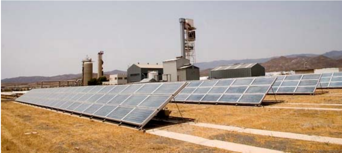
Fig. 3.: 500 m 2 stationary CPC solar collector field
