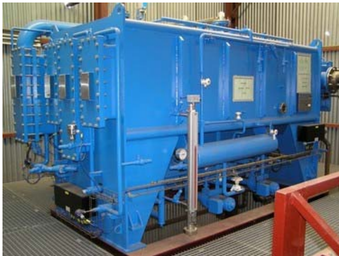
Fig. 7: The new double-effect absorption heat pump installed at the PSA and the energy balance of its coupling to the PSA MED plant
